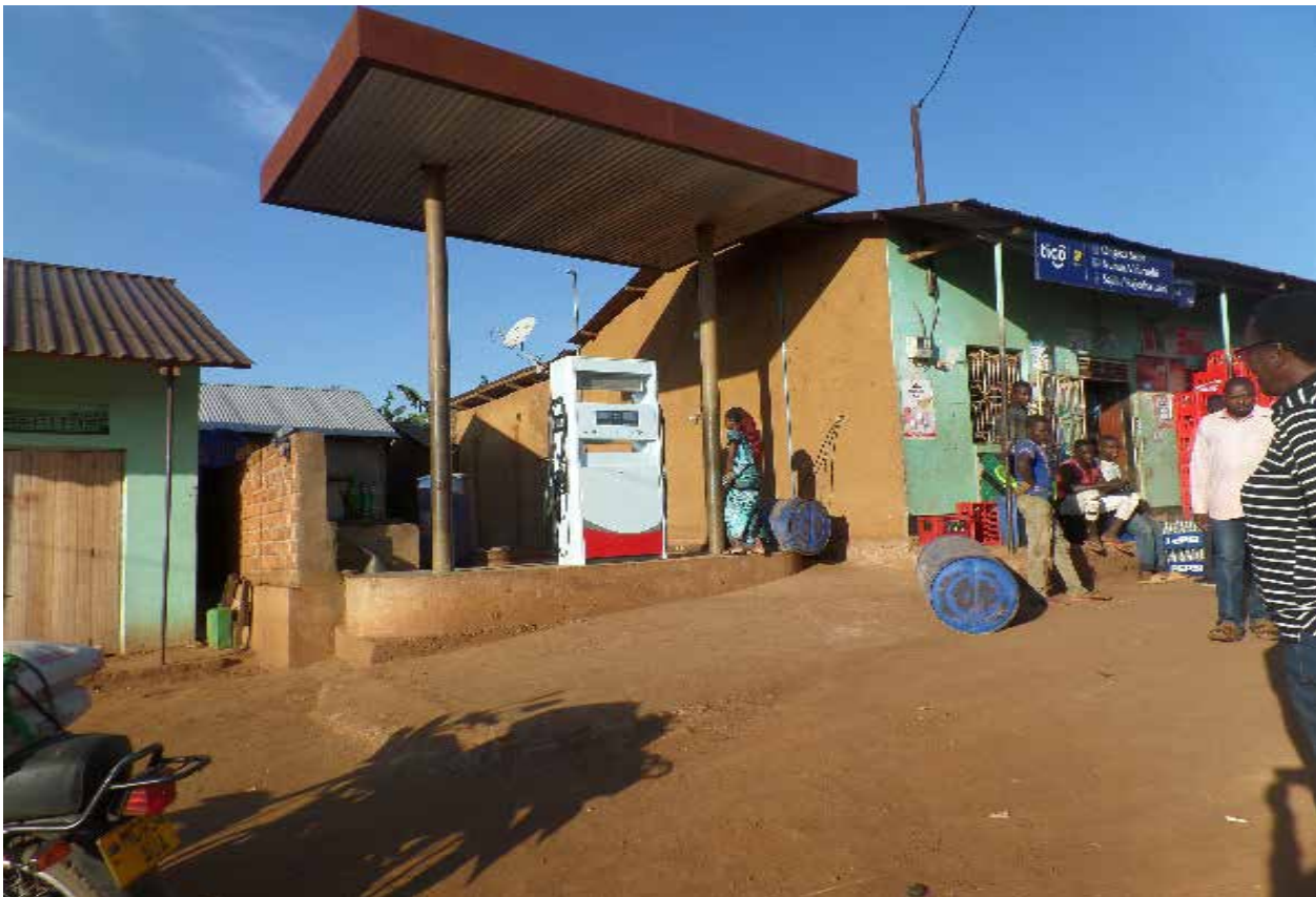
Figure 18: One of the petrol station that is very close to residential houses
