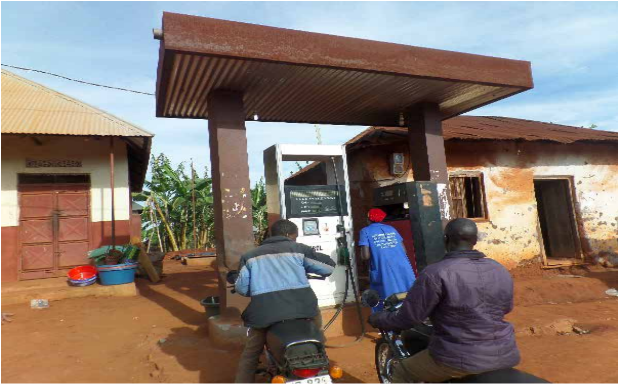
Figure 17: One of the petrol station that is very close to residential houses
